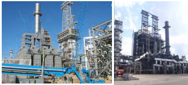
Figure 9. The Frontier Oil Company's (left) and a larger Houston-area refiner's (right) cokers, into whose coker heater tubing C3 has successfully emplaced engineered nanofilms, via in-the-field installation.
